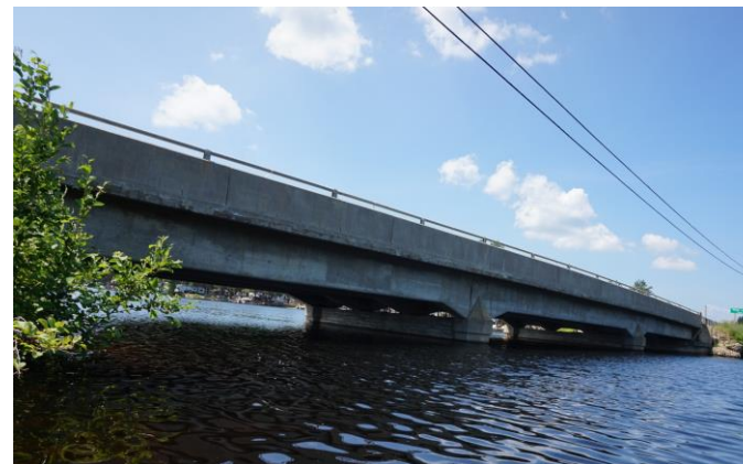
Madawaska River Bridge
