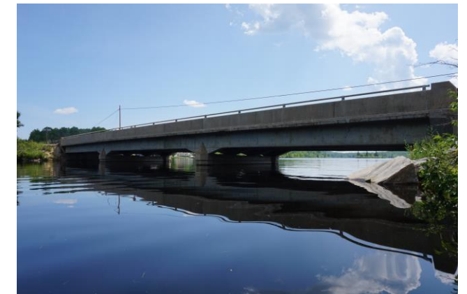
Opeongo River Bridge
