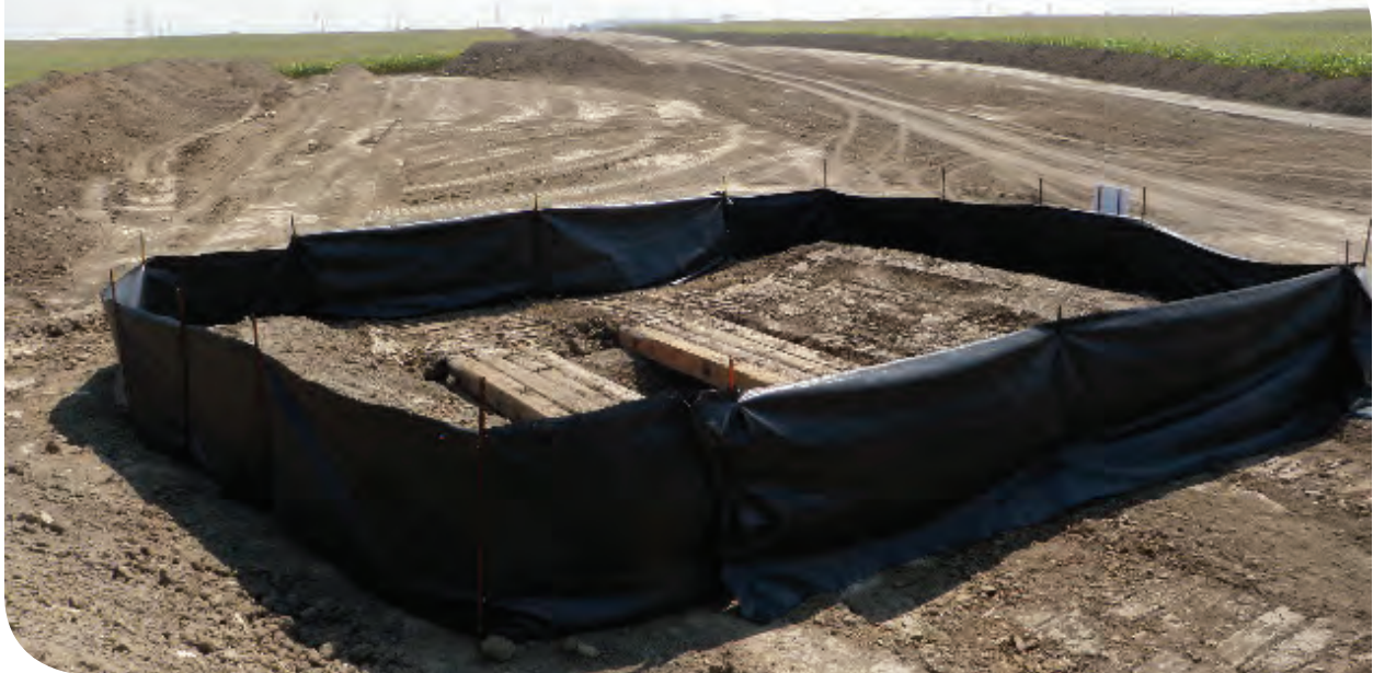
Cleaning station at construction site.
