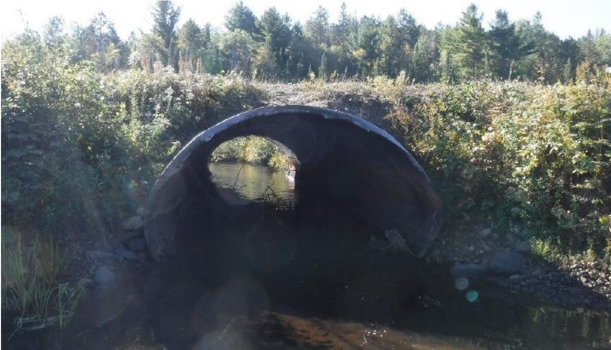
Figure 3-3: Example of Fair Condition Bridge or Culvert – Poverty Creek Bridge
