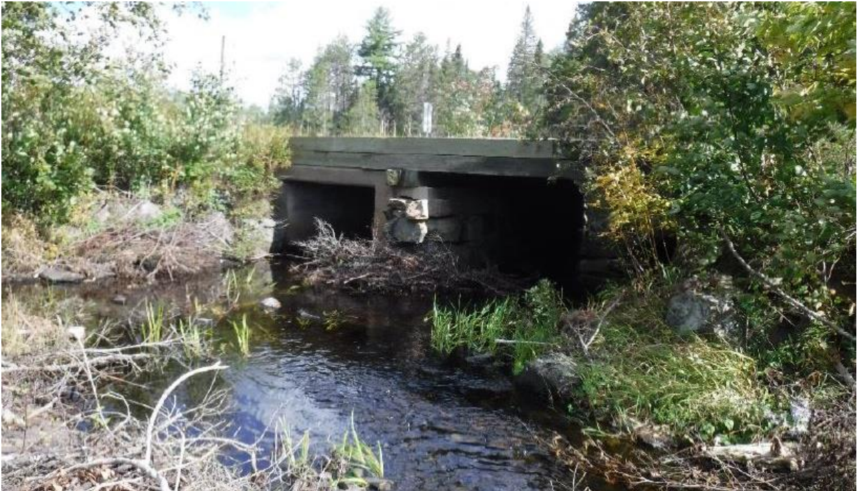
Figure 3-3: Example of Fair Condition Bridge or Culvert – Poverty Creek Bridge
