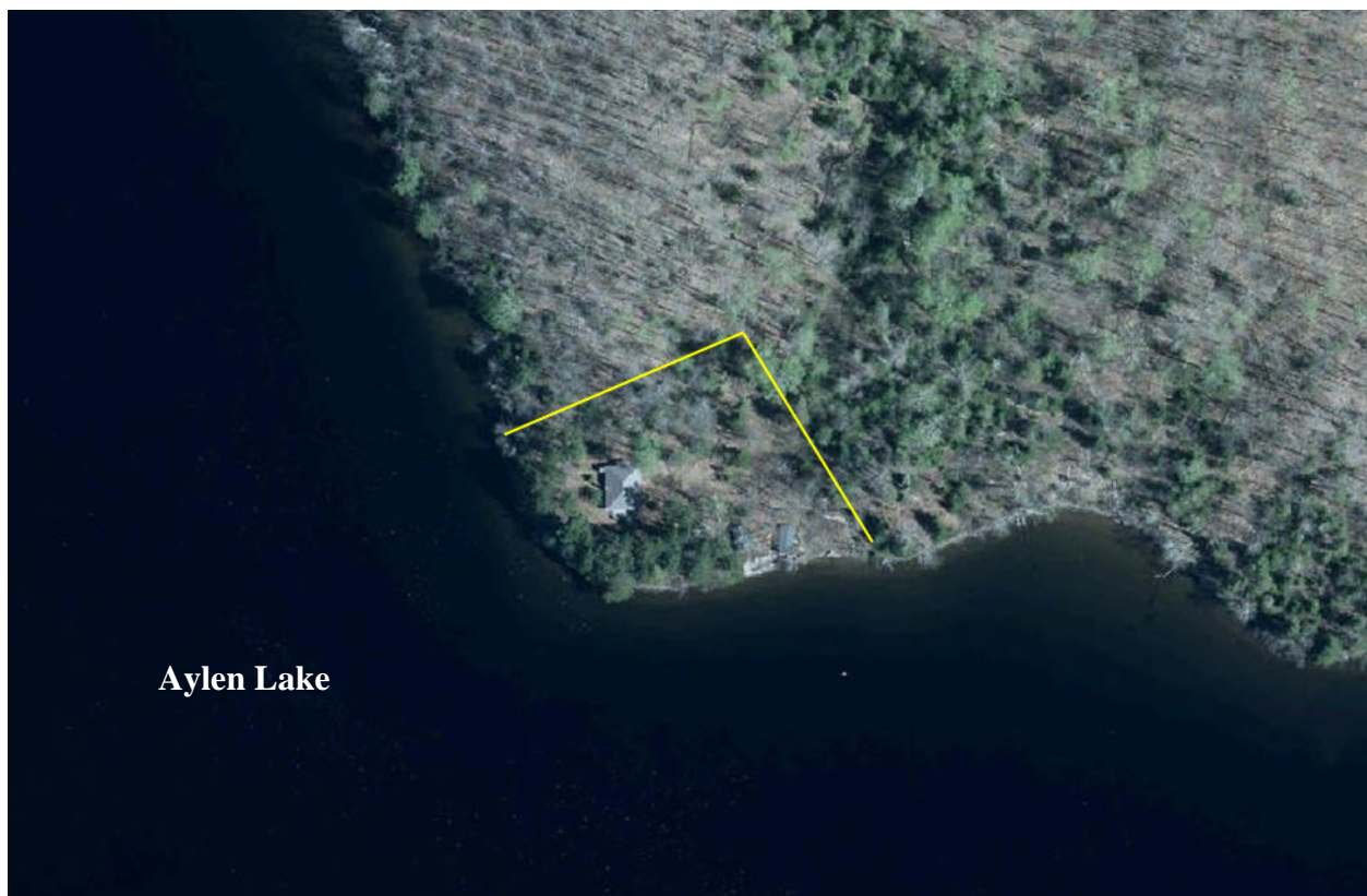
Figure 3 - Property at 1552 Aylene Lake showing location of cottage and outbuildings (image LIO 2020)
