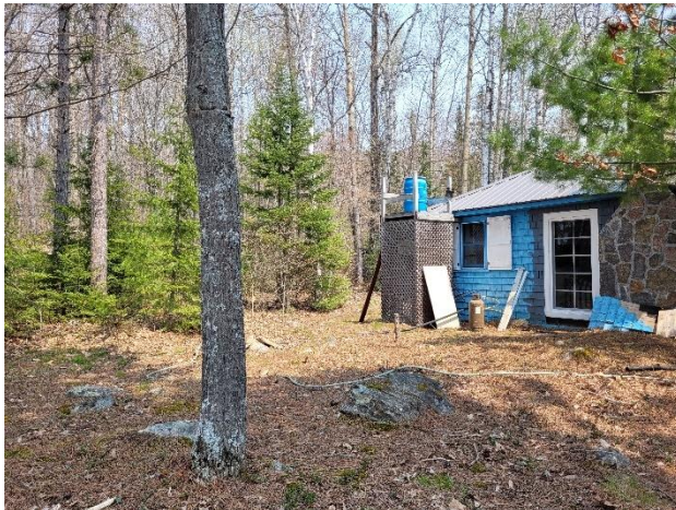
Figure 12 - Cleared area along west side of existing cottage, where proposed addition is to be constructed (8 May 2023)
