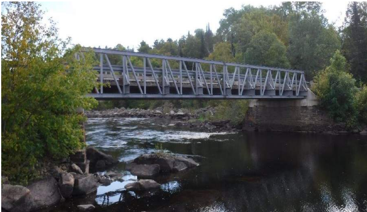
Figure 3-4: Example of Good Condition Bridge or Culvert – Algonquin Street Bridge
